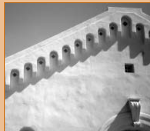
Original diamond shaped tiles on the temple façade have been excavated and restored, July 30th
