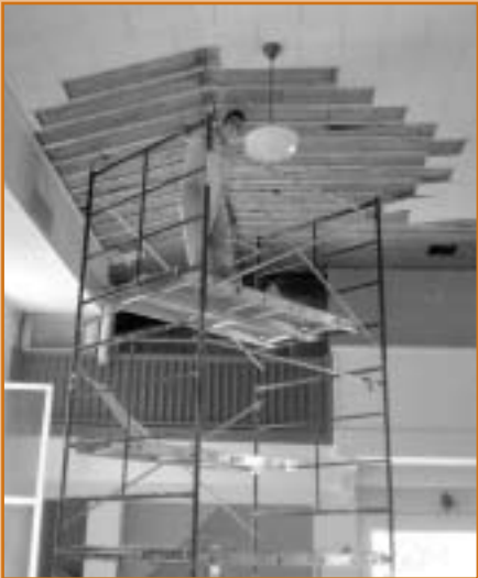
Worker begins removing ceiling tiles in temple sanctuary, June 18th
