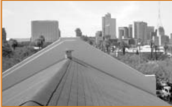
The heritage center sports a brand new roof, July 30th
