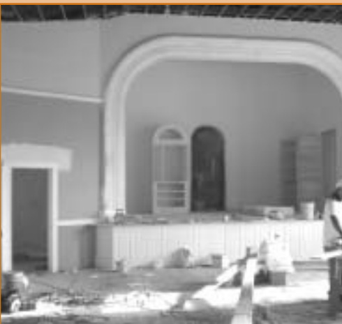
Workers restore sanctuary interior, August 8th
