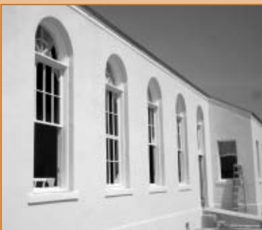
Restored exterior windows are reinstalled, July 31st
