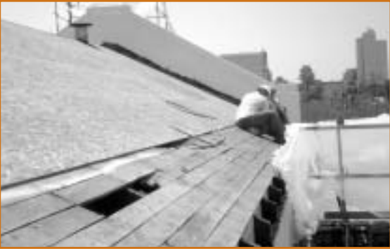
Workers install new decking on roof, July 3rd
