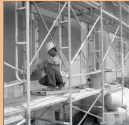
Worker applies new stucco to exterior, July 14th
